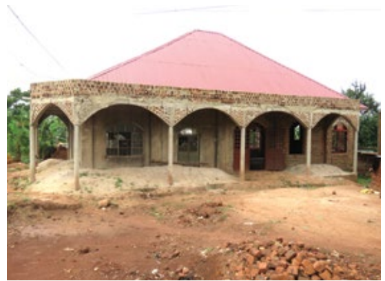
Re-construction and renovation of Masjid Taqwa - Kijabijjo.
